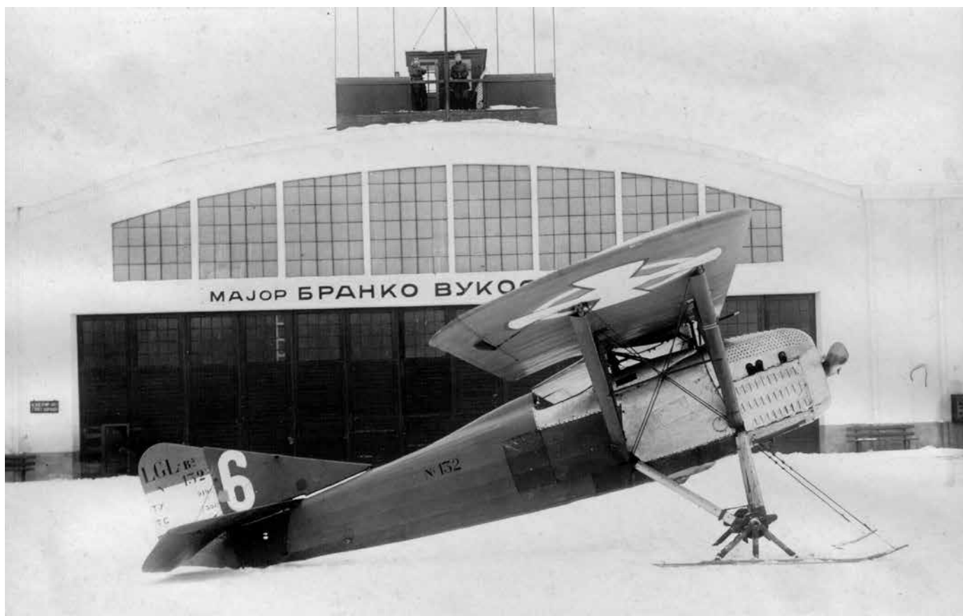
A modification frequently used on VV KSHS aircraft in winter months: Loire-Gourdou-Leseurre B3 no.132 of 1.VP with built-in skis at Novi Sad aerodrome.
